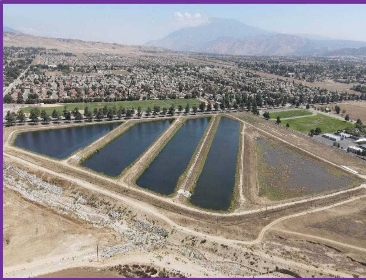
Brookside East Recharge Facility
