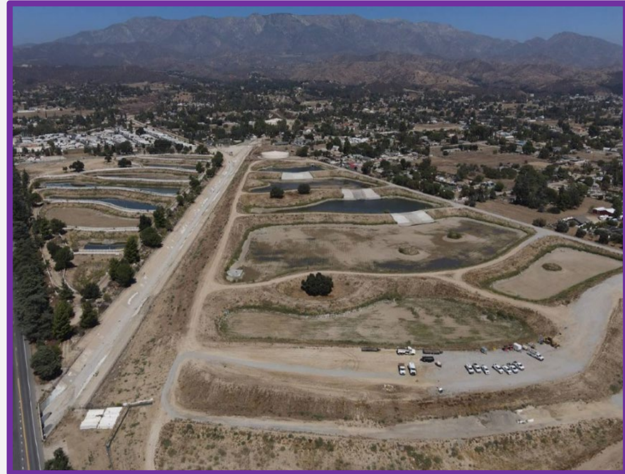
BCVWD Recharge Facilities
