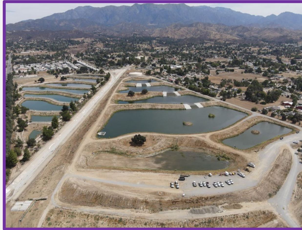
BCVWD Recharge Facilities
