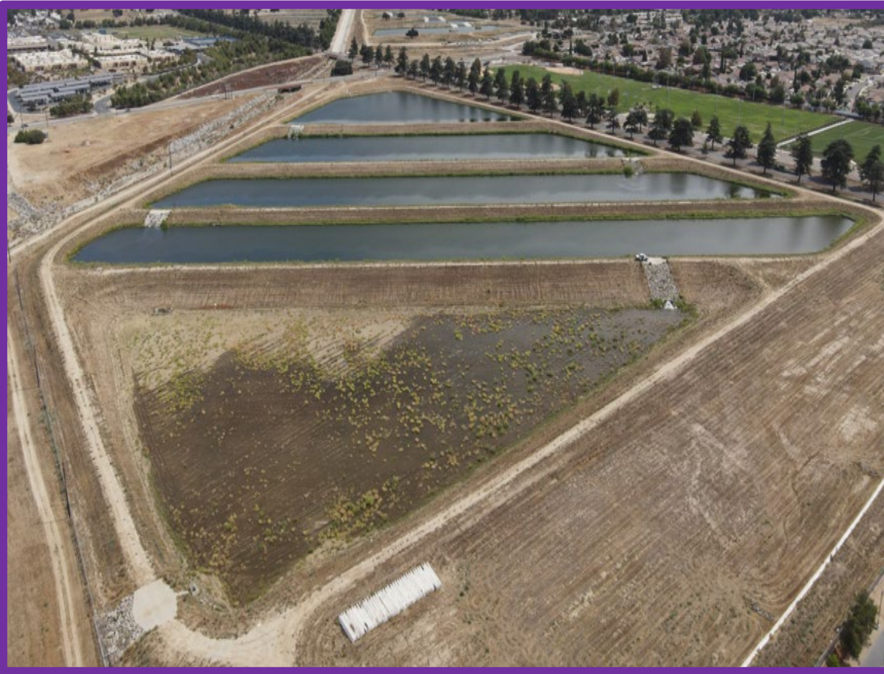
Brookside East Recharge Facility
