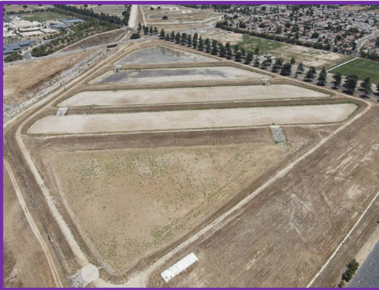
Brookside East Recharge Facility
