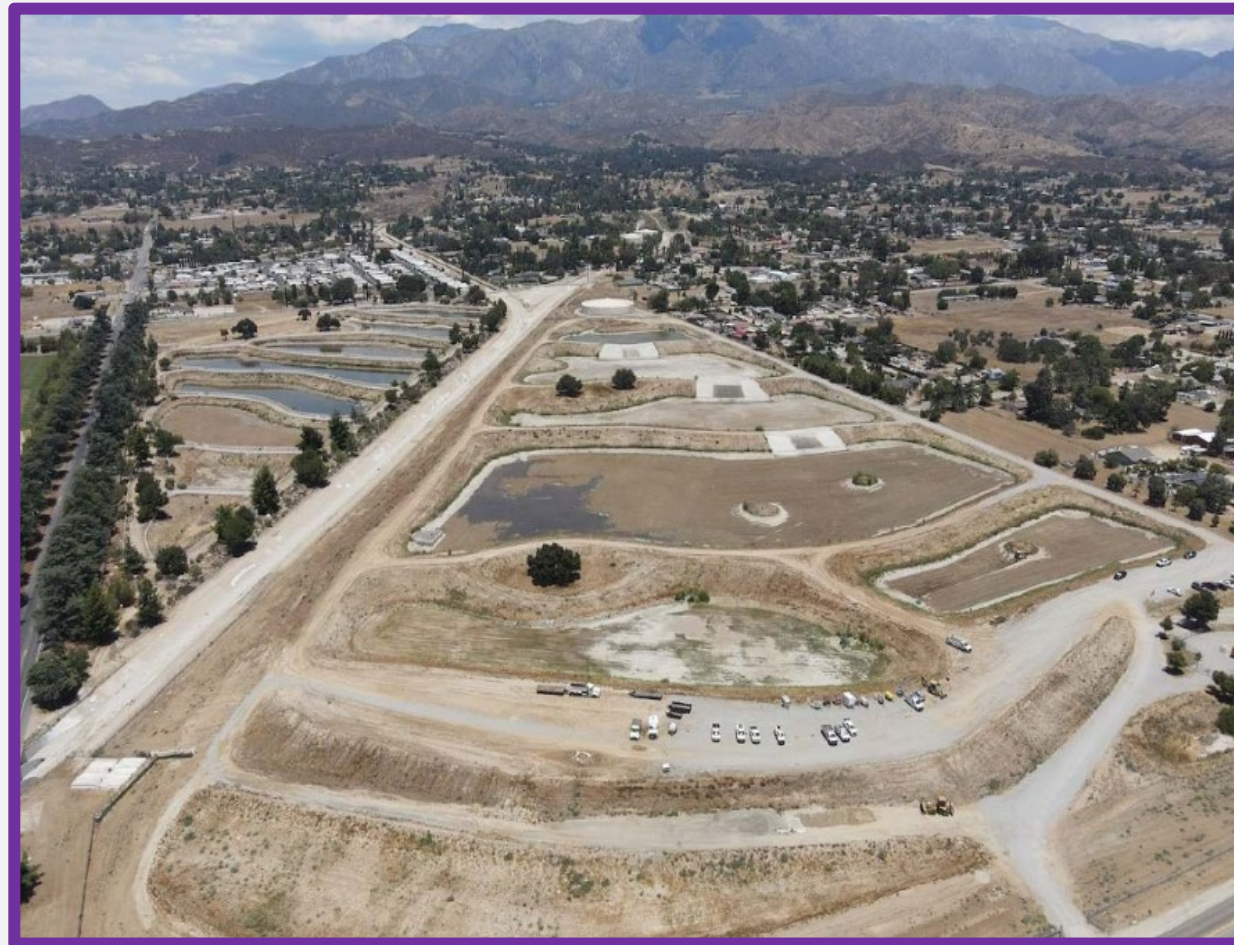
BCVWD Recharge Facilities
