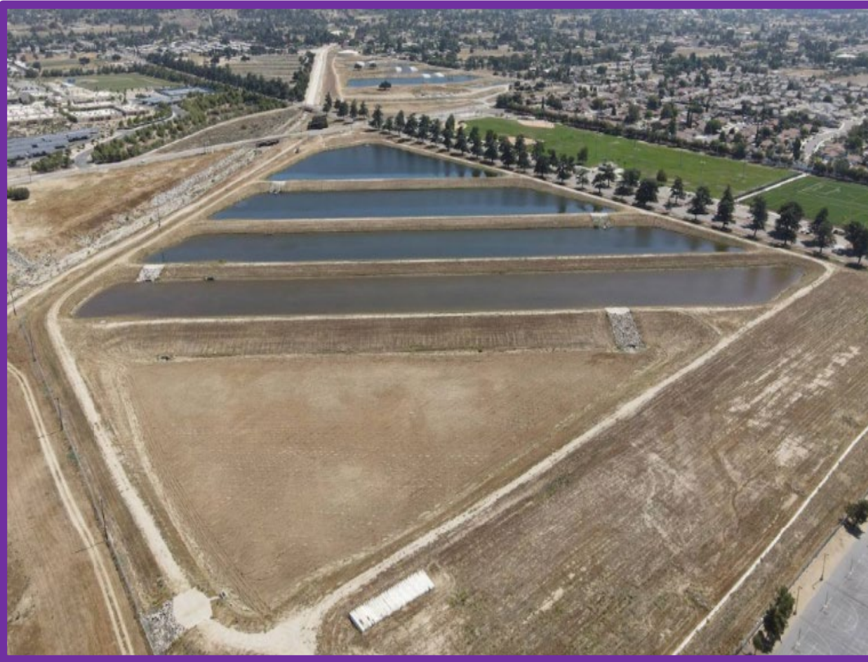
Brookside East Recharge Facility
