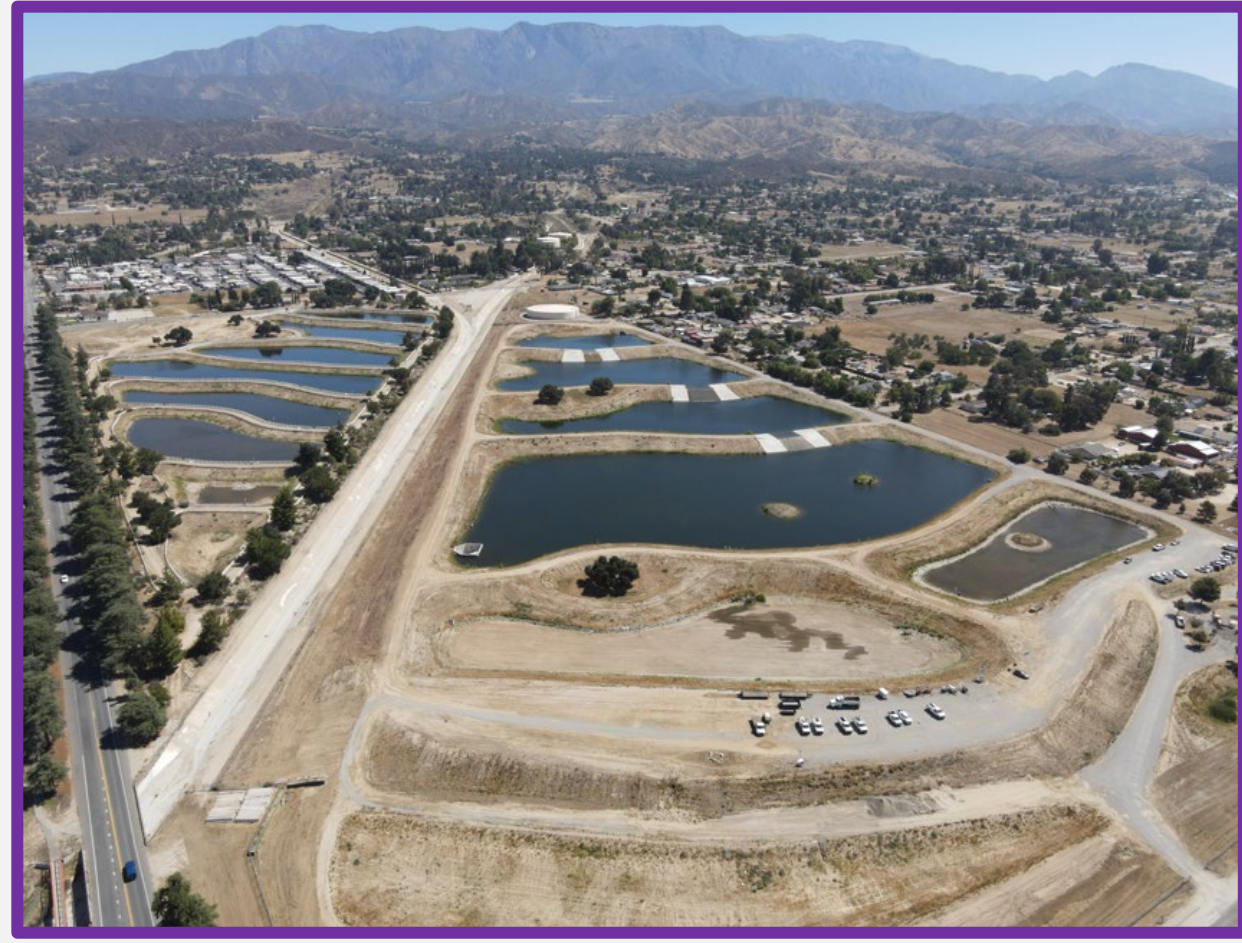
BCVWD Recharge Facilities
