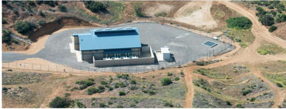
Cherry Valley Pump Station
