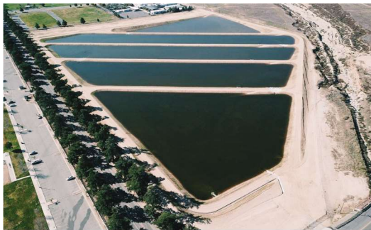
Brookside East Recharge Facility
