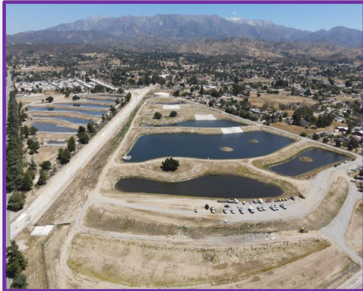
BCVWD Recharge Facilities
