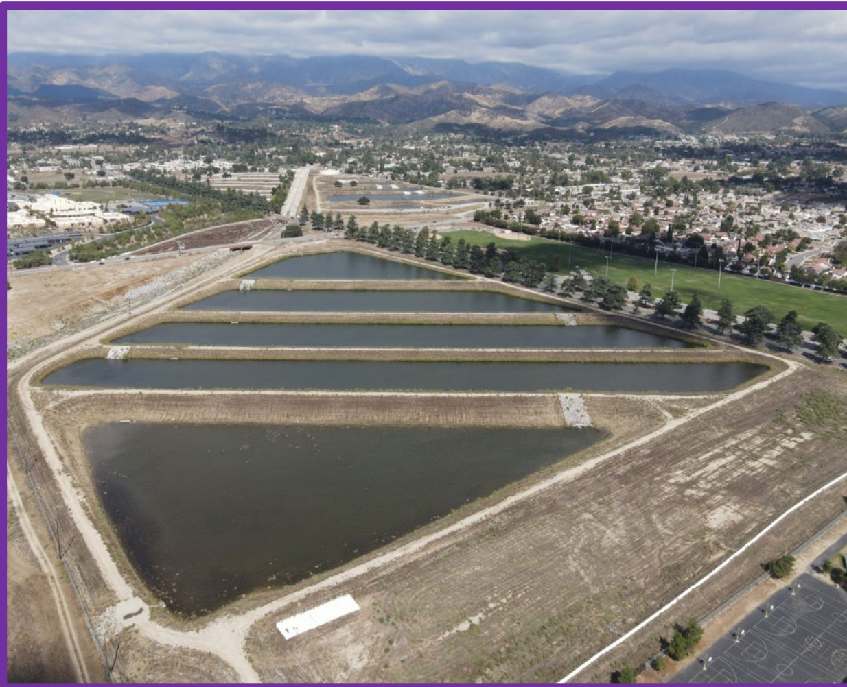
Brookside East Recharge Facility
