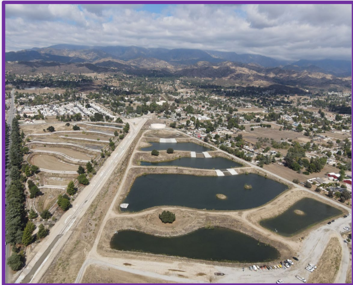
BCVWD Recharge Facilities
