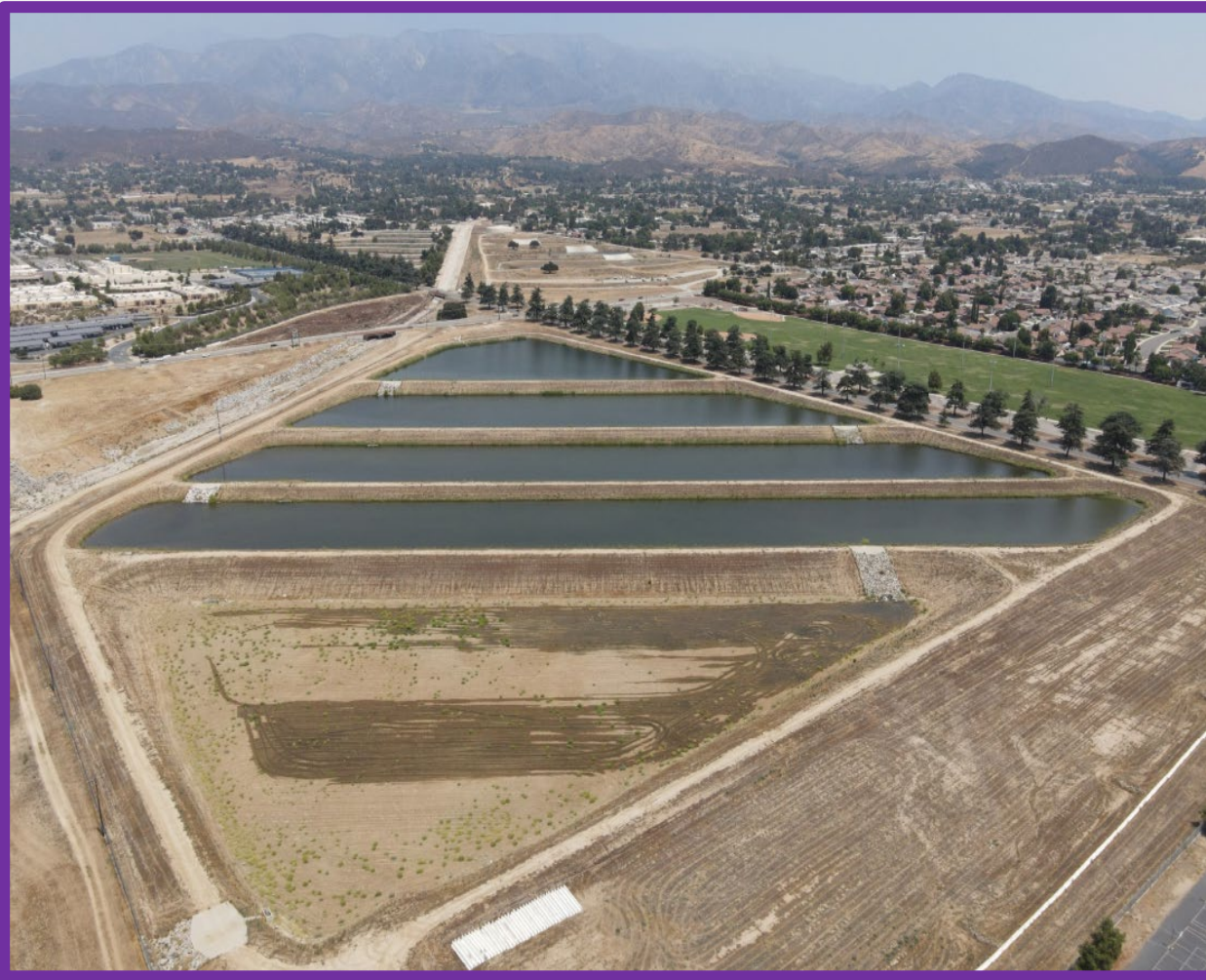
Brookside East Recharge Facility
