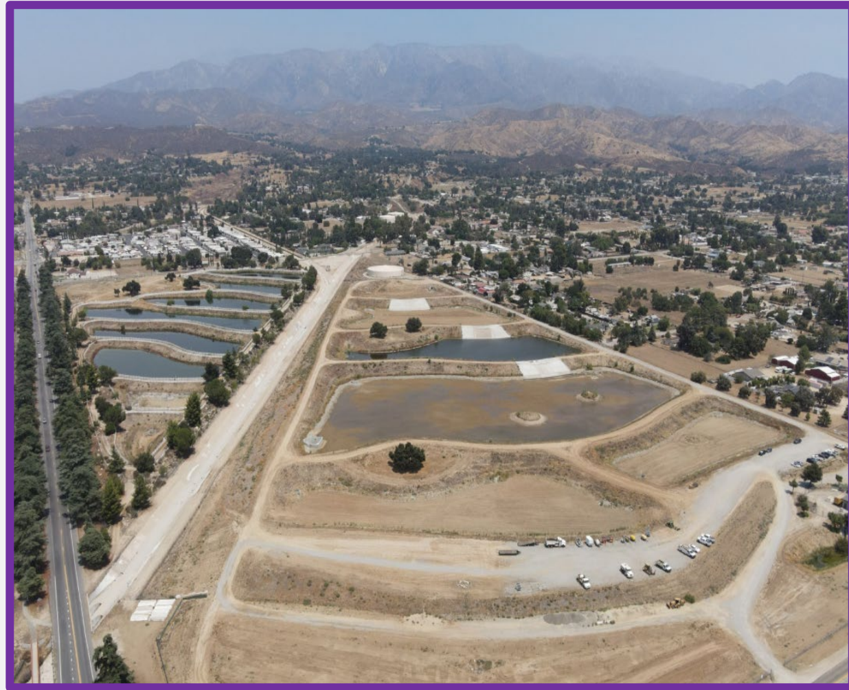
BCVWD Recharge Facilities
