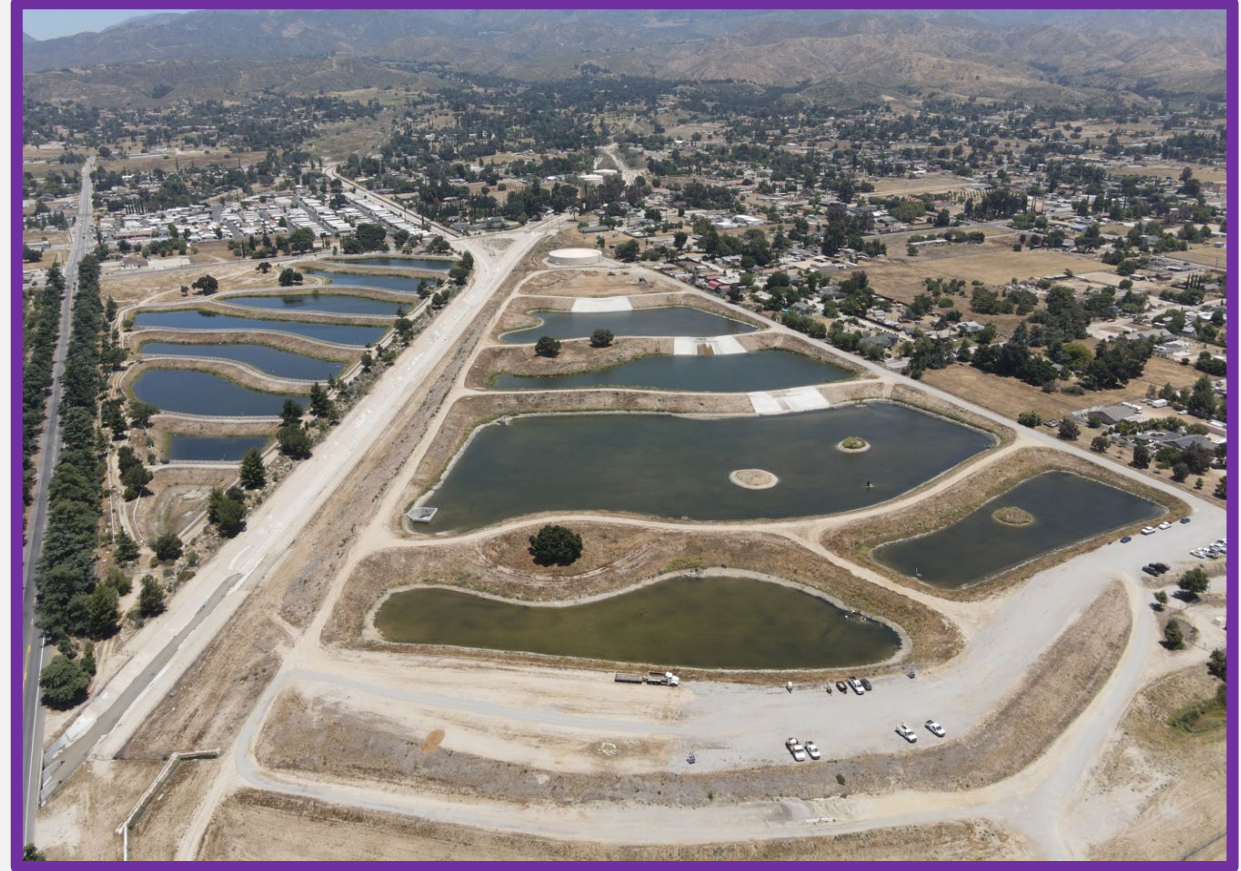
BCVWD Recharge Facilities
