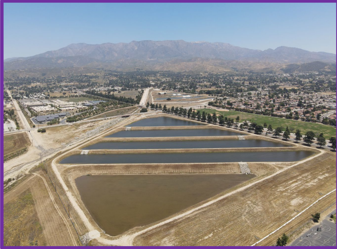
Brookside East Recharge Facility
