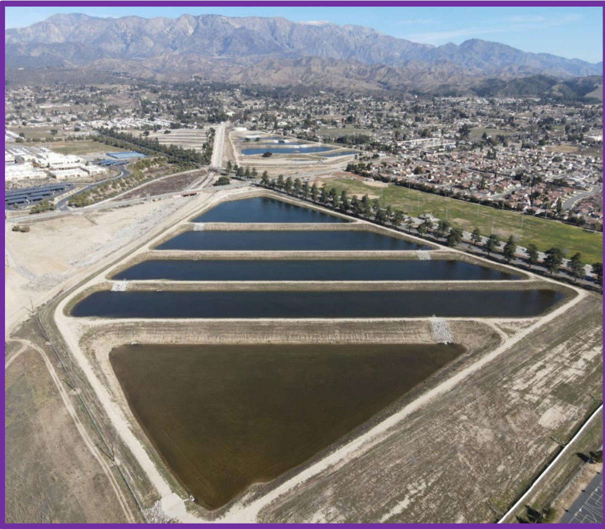
Brookside East Recharge Facility
