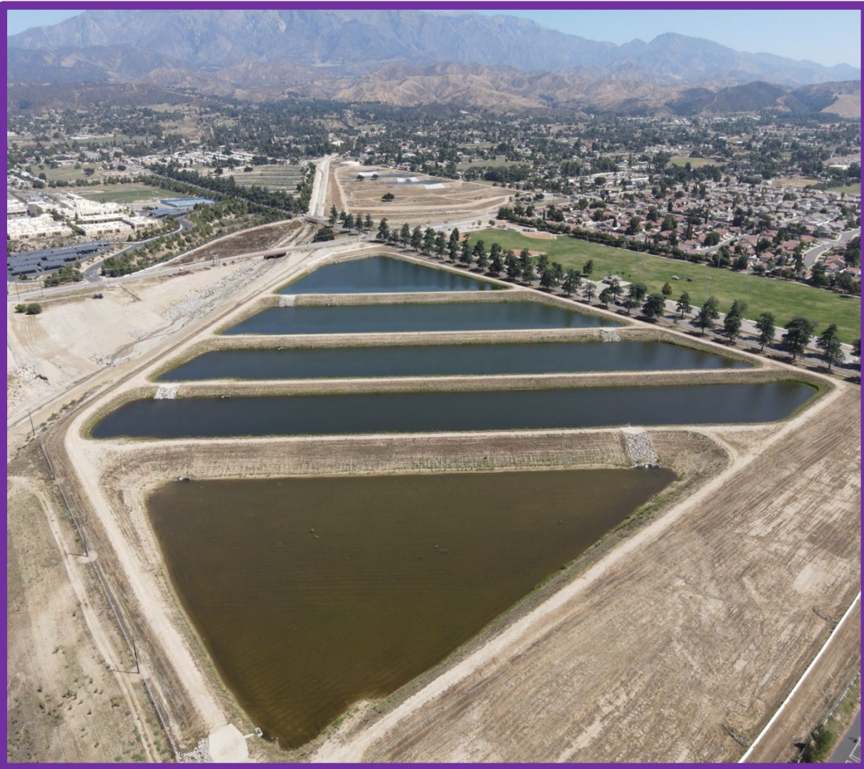
Brookside East Recharge Facility
