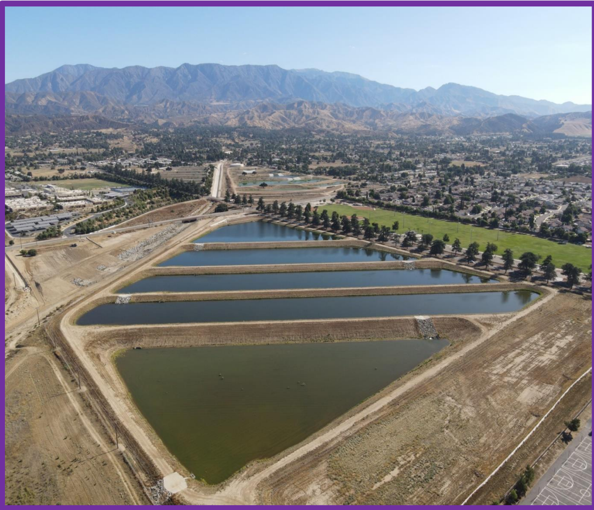
Brookside East Recharge Facility
