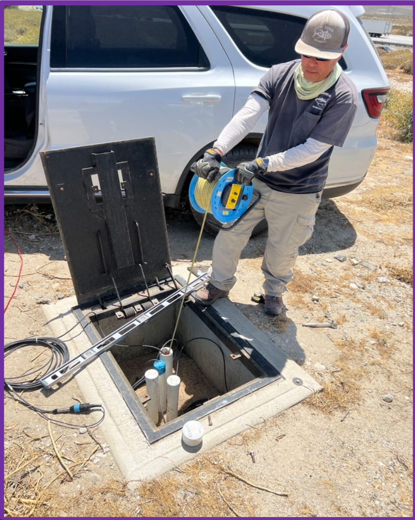
USGS Measuring Monitoring Well
