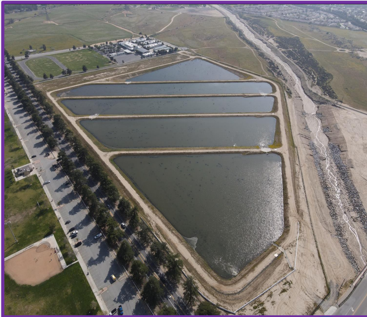
Brookside East Recharge Facility
