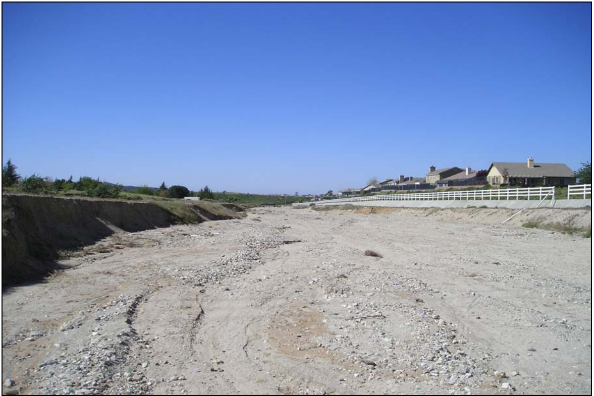
Photograph 3: Overview of the eastern bank of Noble Creek. View to the south-southwest.
