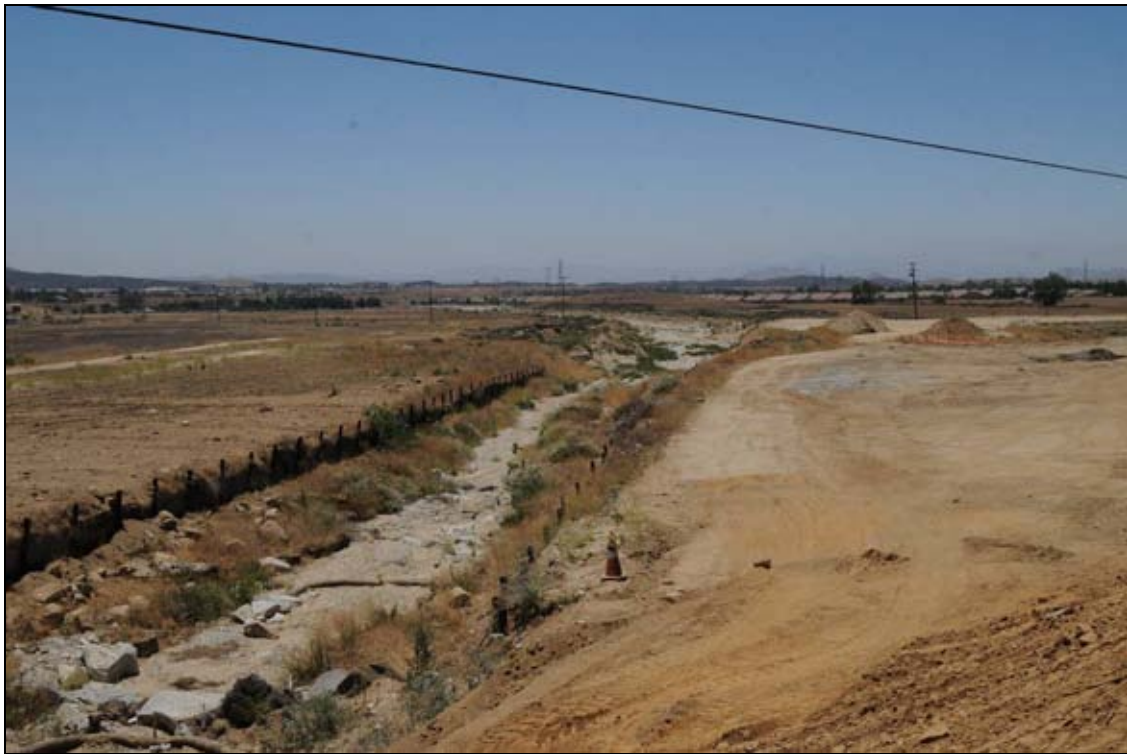
Photograph 1: Looking south (downstream) from Beaumont Avenue showing Noble Creek.
